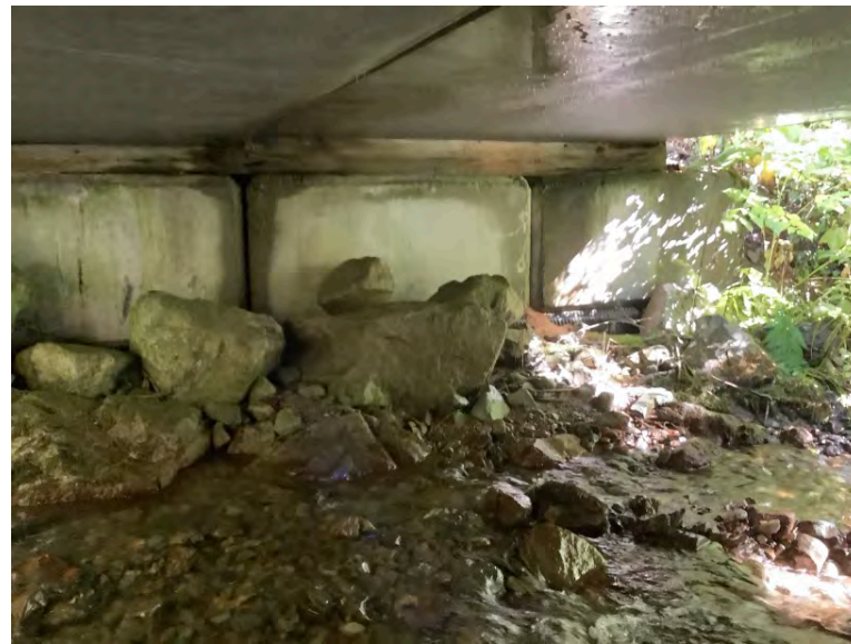
Left Bank Abutment when facing downstream
