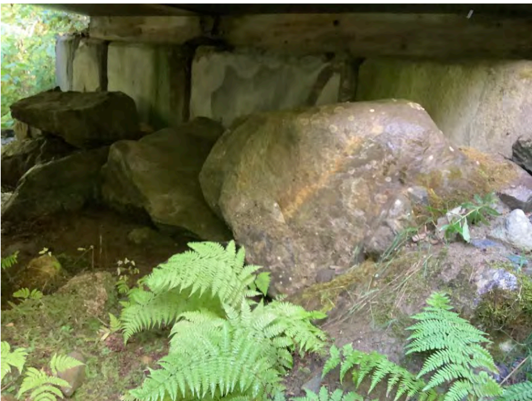
Right Bank Abutment when facing downstream
